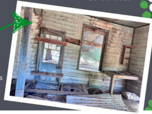
The remains of the old Schoolhouse
